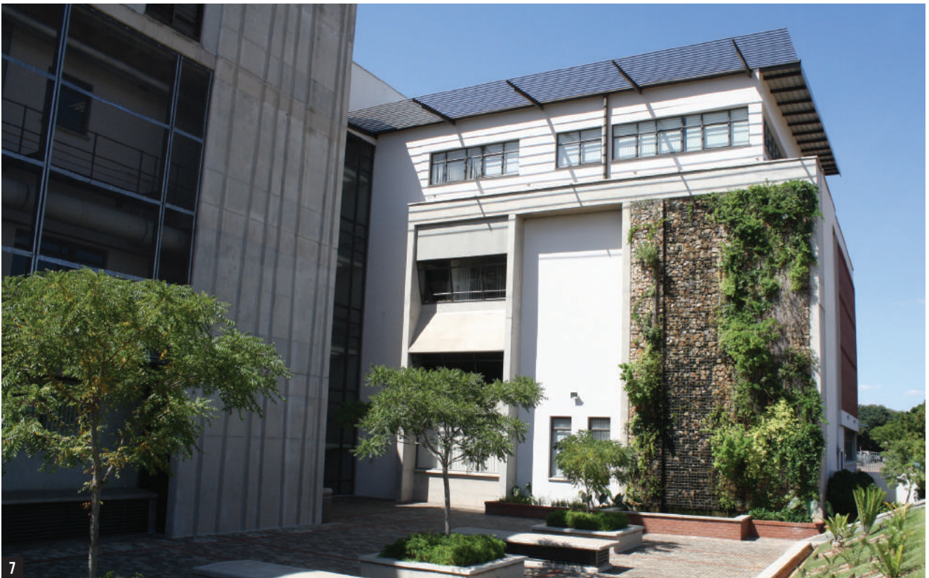
7 The west facing wet living wall of the UP Plant Sciences building (image by author).
