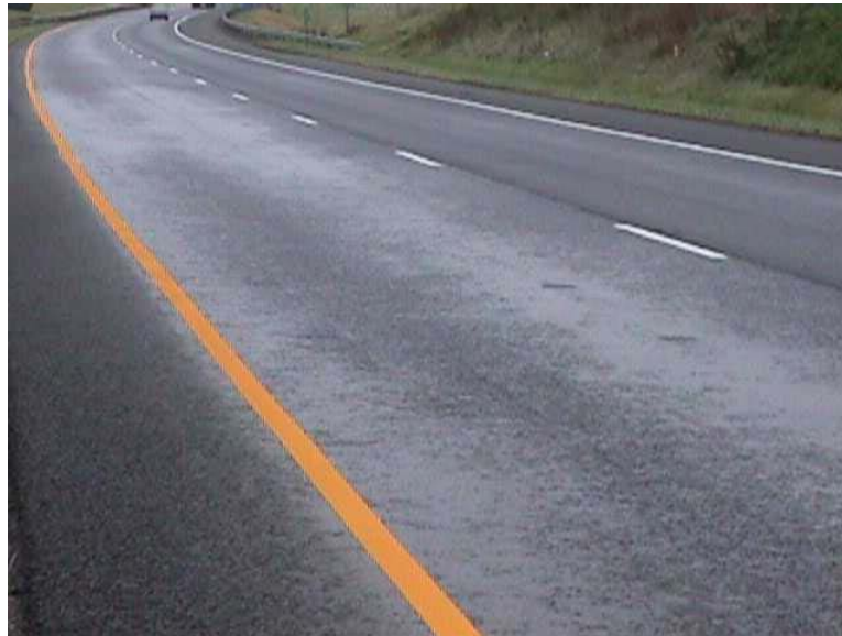
Picture 2. Flushing Due to Wet Mineral Filler.
