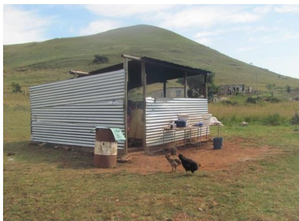
Photograph 4.9: A shelter construction for preparation of food for students daily
