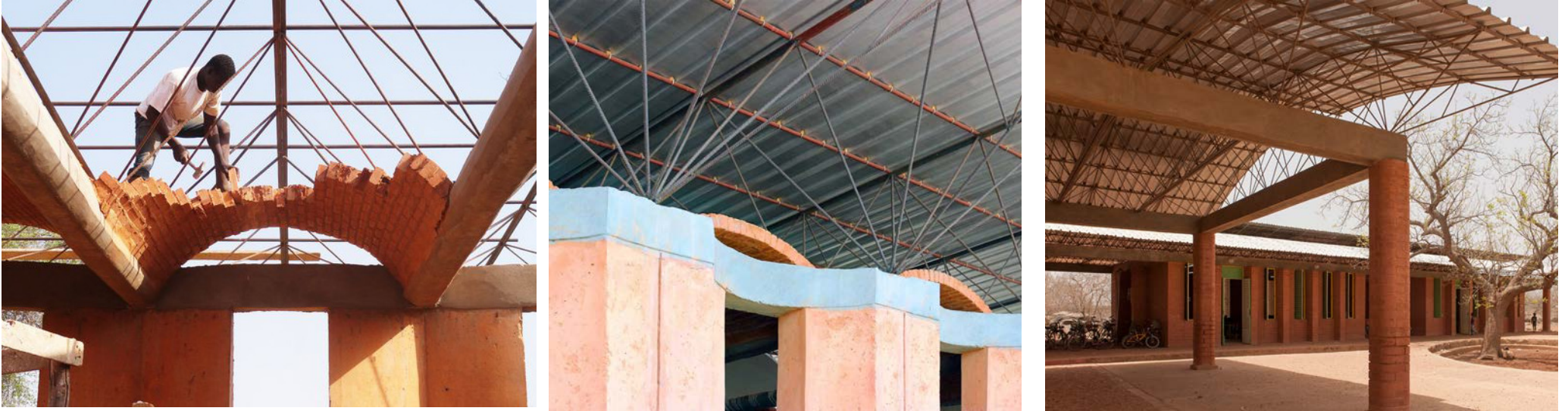
Fig 8.22 Double roof construction, Picture, Francis Kere, Laongo Opera Village (2016)
