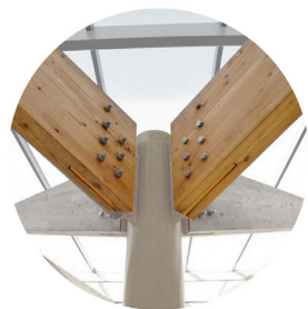
Laminated timber beams as secondary and tertiary structure.
