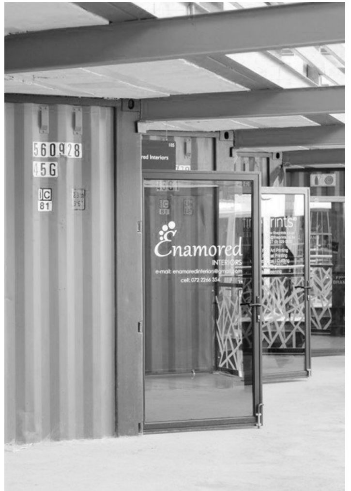
Figure 4.12 Spatiality and Construction (27 Boxes 2015)
