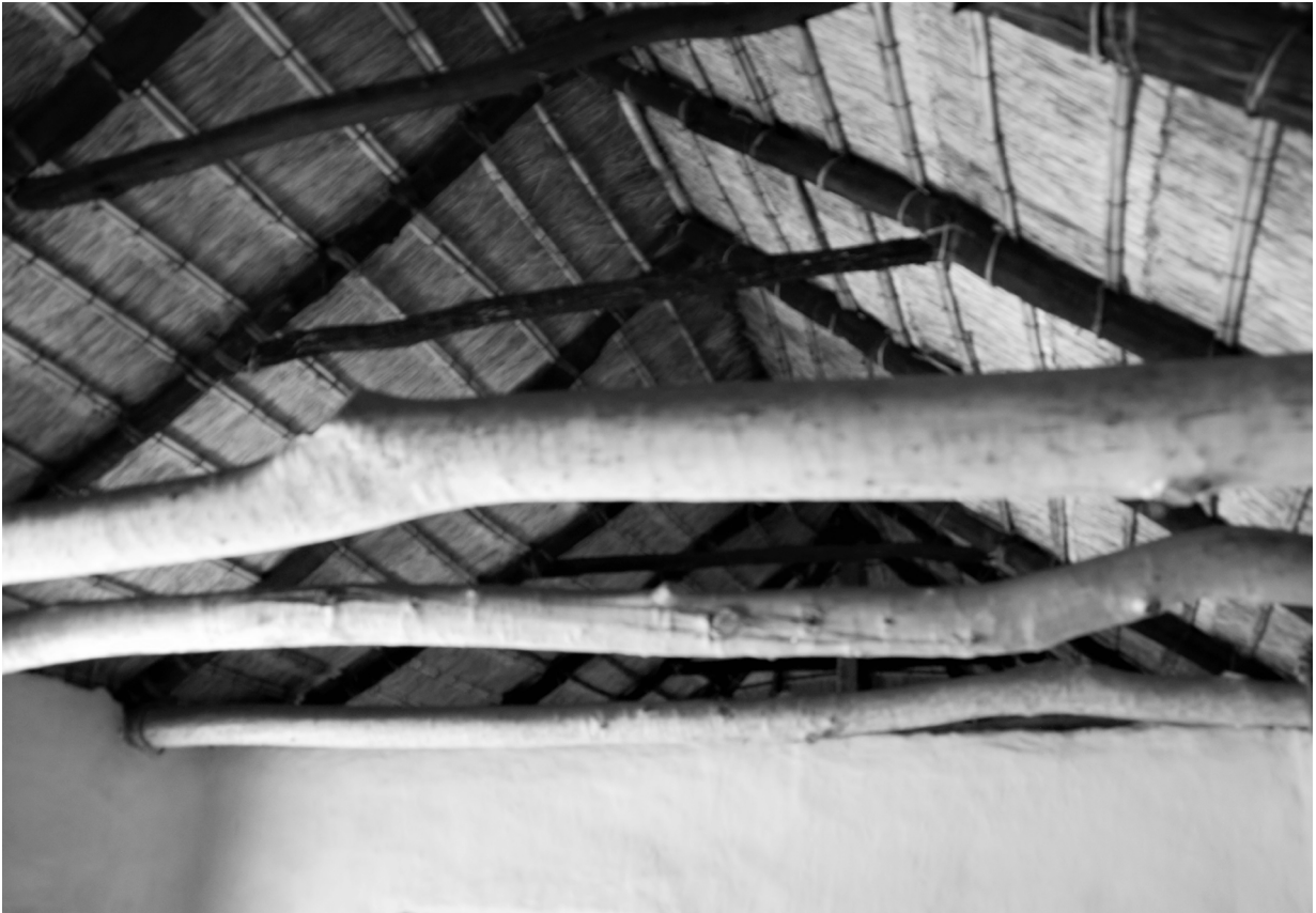
Figure 3.10 Construction of the Pioneer House (Author)
