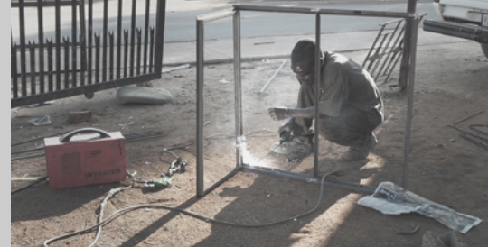
Figure 1.17 Sidewalk as “welding booth”(Author, 2016)
