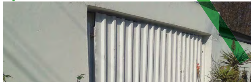
FIGURE 196 Perspective of the eastern entrance for waste delivery. Images making reference to the suburban garage door, to the right a plan displaying movement of waste from waste entry and finally a precedent of movement with the SpielbudenPlatz project by NL Architects/ http://www.gkdmalfabrics.com/files/news/big/da7ab74cb3a1a7163fd98d2f9223b228.gif
