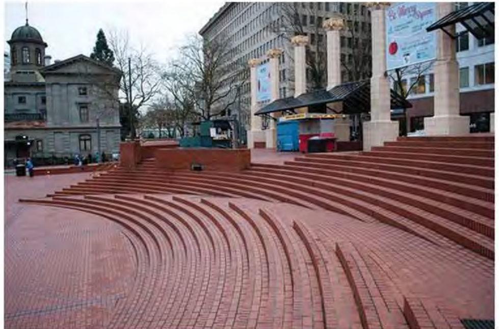
PRECEDENT , Cory Silva masonry ramp stair design
