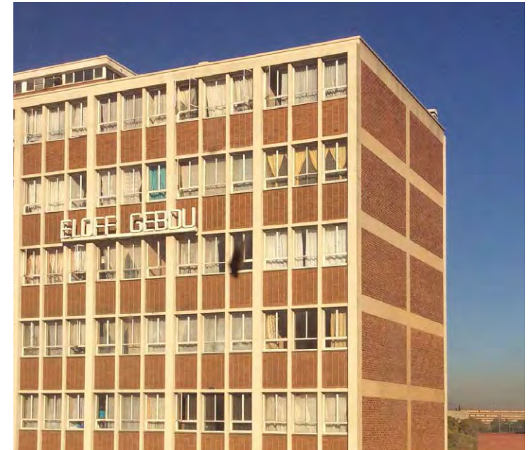
Figure 102 Building opposite site used as an example to show structure as an expressed element on the façade and the gabion wall in-filled with brick.
