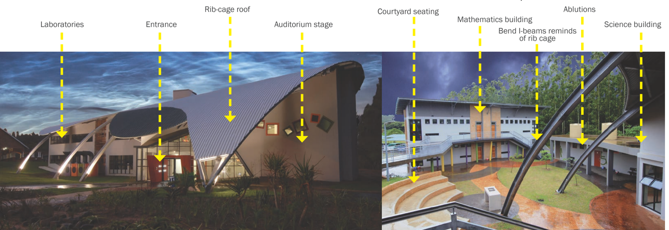
Figure 4.8 Photo looking north-west of Science building (TJA)
