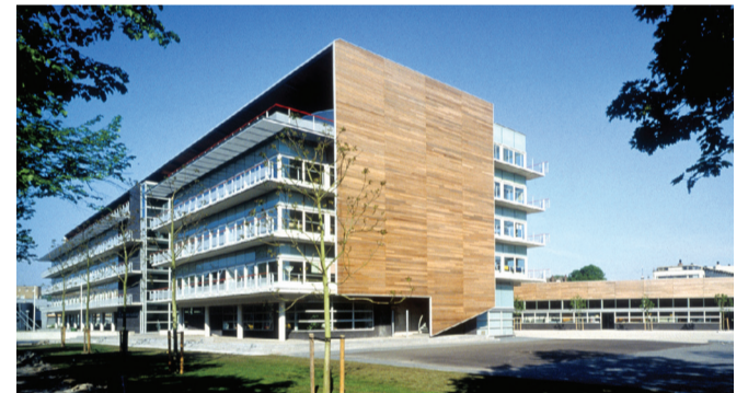
Figure 4.25 Photo of school building exterior (Unknown)
