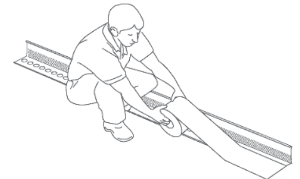
Taping an aluminium edge to an EPDM rubber membrane
