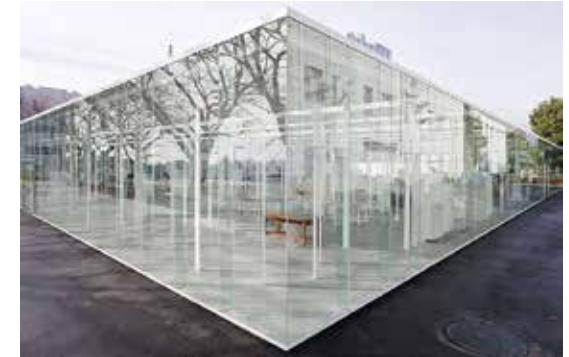
Figure 9.12 (Junya Ishigami + associates, 2008)
