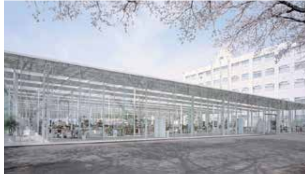
Figure 9.11 (Junya Ishigami + associates, 2008)
