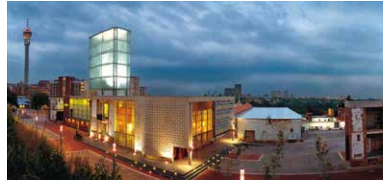
Figure 4.18 The completed Constitution Hill Precinct (Constitution Hill, 2015)
