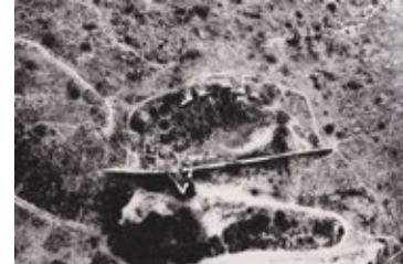
Figure 2.6: Fort Wonderboompoort after construction (Van Vollenhoven:1996)
