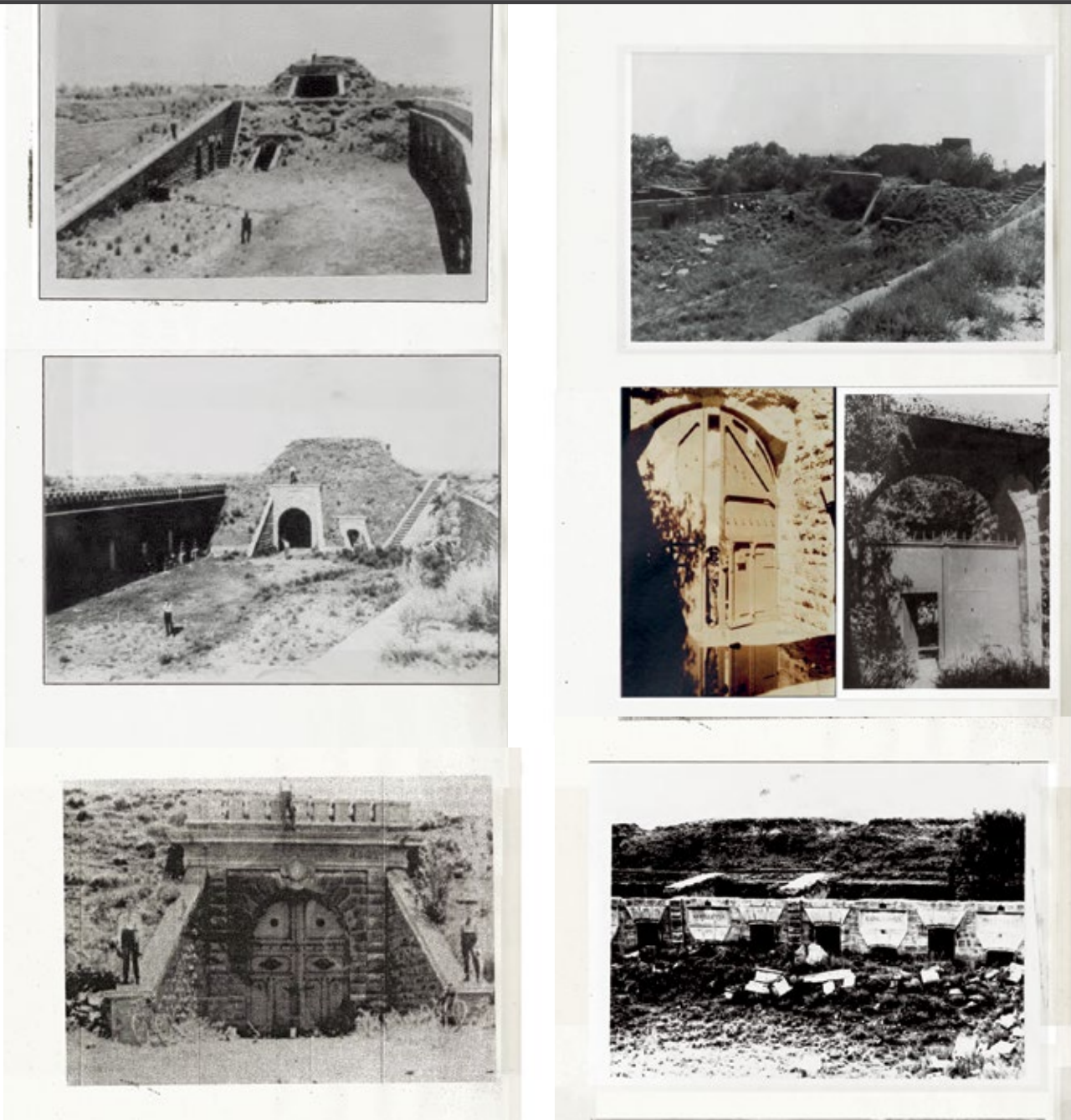
Figure 2.9: Fort Daspoortrand after construction (Van Vollenhoven:1996)
