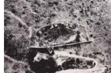
Figure 2.6: Fort Wonderboompoort after construction (Van Vollenhoven:1996)
