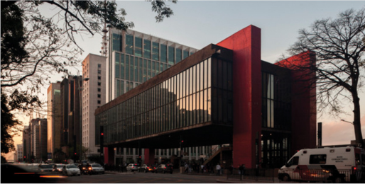
FIGURE 5.2 MASP Photograph of MASP from the street looking towards the public plaza space
