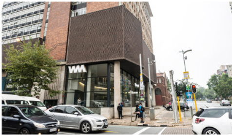
FIGURE 5.15 NEW DEFINED STREET EDGE Photograph depicting the new layer attached to the facade used to define the street edge
