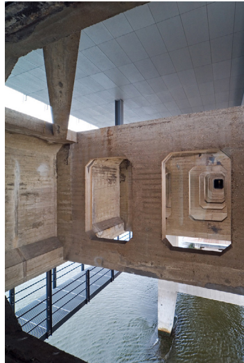
Fig 4.14 view from below the Kraanspoor building (Archdaily, 2008).
