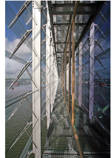
Fig 4.17 Double glazing panels with louvres of Kraanspoor building (Archdaily, 2008).
