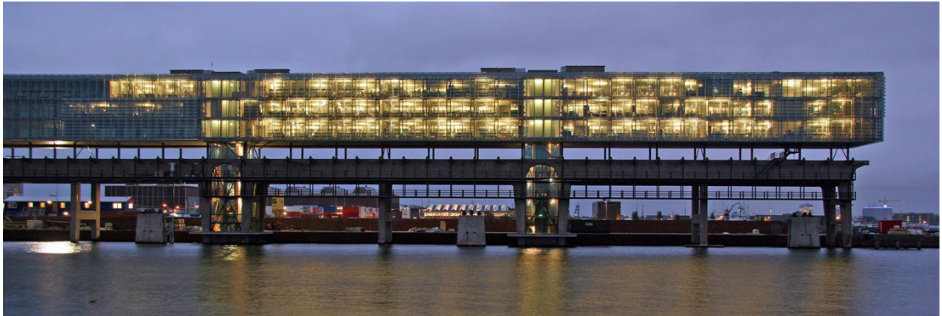
Fig 4.18 View from water of Kraanspoor building sitting lightly above existing historical structure. archdaily. 2008.
