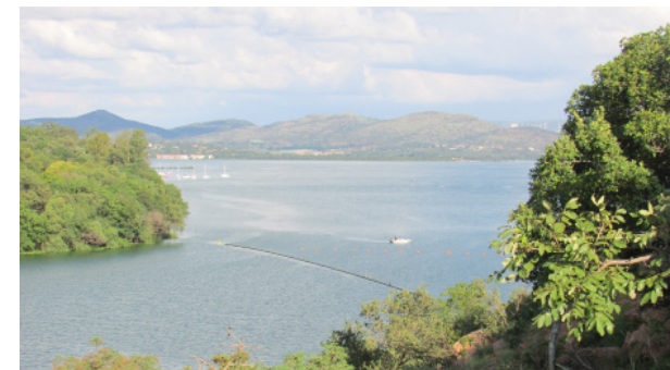
Fig 2.21 The dam today (Author, 2016).
