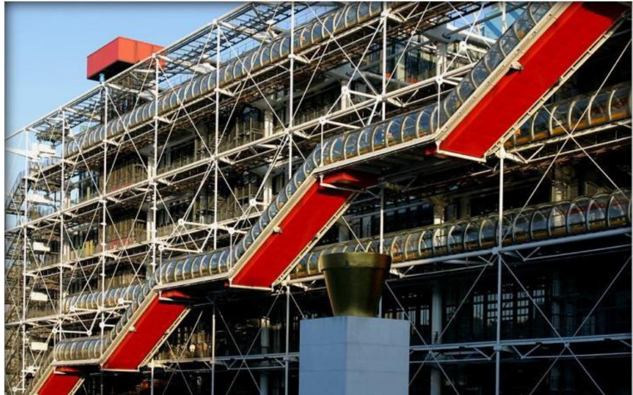
Fig 5.15 Services and circulation of the facade of the building (Archdaily, 2016).
