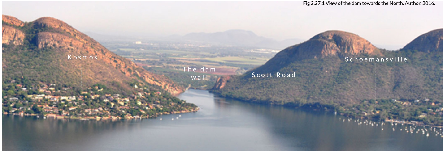
Fig 2.27.1 View of the dam towards the North. Author. 2016.
