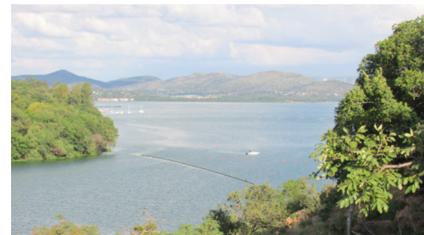
Fig 2.21 The dam today (Author, 2016).
