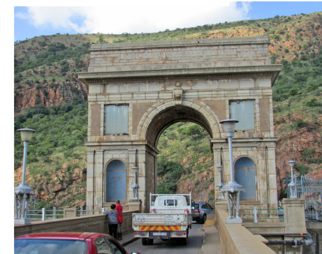
The Arch Fig 2.25 the Arch at Hartbeespoort dam (Author, 2016).
