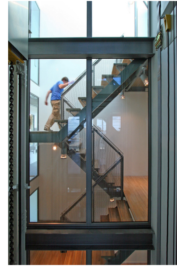
Fig 4.16 New stairway up Kraanspoor building (Archdaily, 2008).
