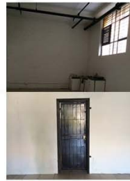
Existing window and steel door which open up onto the courtyard
