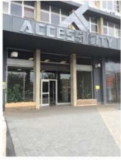
OFFICE SPACE industrial fabric, exposing materiality
