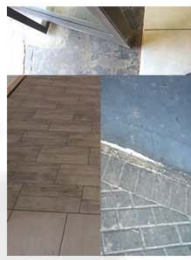
Floor finishes: neutral tiles and painted concrete screed
