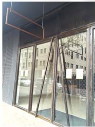
Steel shopfront doors, retail opportunity
