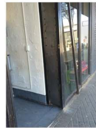
Steel door frame to plastered brick wall
