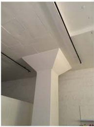
Interior columns: footing at soffit, plastered, white
