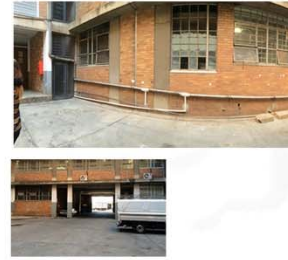
Accesspoint into the courtyard, towards the wall of site from within the courtyard
