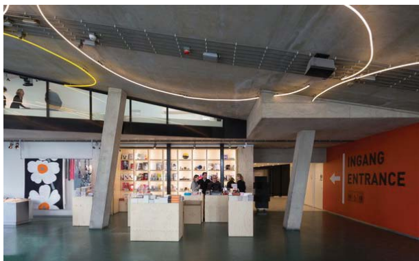
Figure 10.15 ~ Kunsthal slanted columns.jpg Kunsthal Rotterdam. Photo indicating the slanted columns in response to the ramped floor above. Source: OMA
