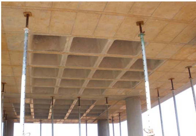
Figure 10.9 ~ DBSA coffer slab.jpg The roof structure, a reinforced concrete coffer slab. Source: HolmJordaan
