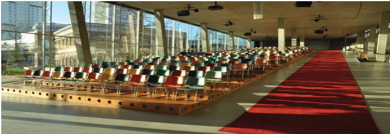
Figure 10.14 ~ Kunsthal slanted columns auditorium.jpg Kunsthal Rotterdam. Photo indicating the slanted columns in response to the ramped floor above. Source: OMA
