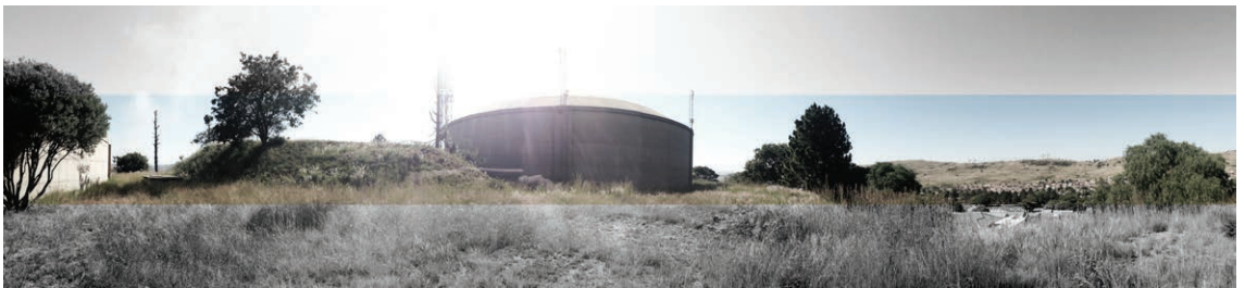
Fig. 71. Atteridgeville Reservoir - north.
