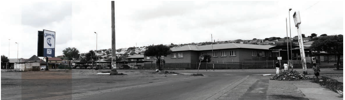
Fig. 46. Southern view of Atteridgeville Clinic on Ramohoebo
