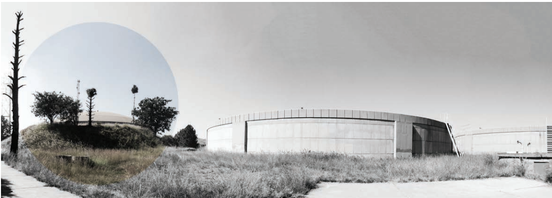
Fig. 68. Atteridgeville Reservoirs - south-east.
