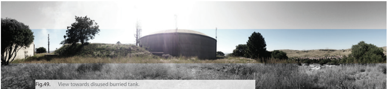
Fig.49. View towards disused buried tank.
