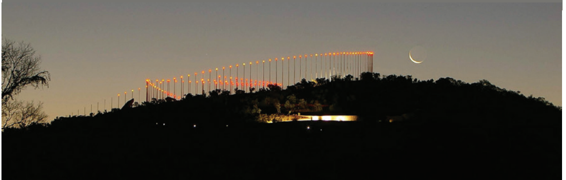
Fig.55. The Freedom Park. Southern Elevation, Architecture is noticeable in the Reed lights at dusk. Graham A. Young, 2012.
