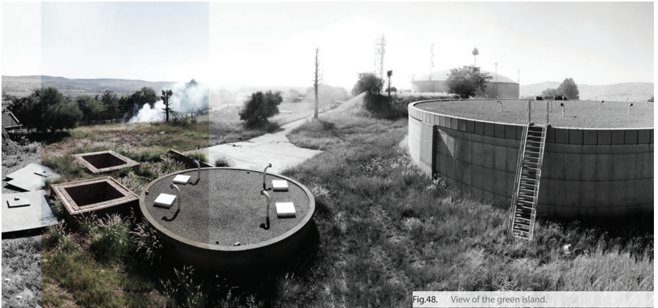
Fig.48. View of the green island.
