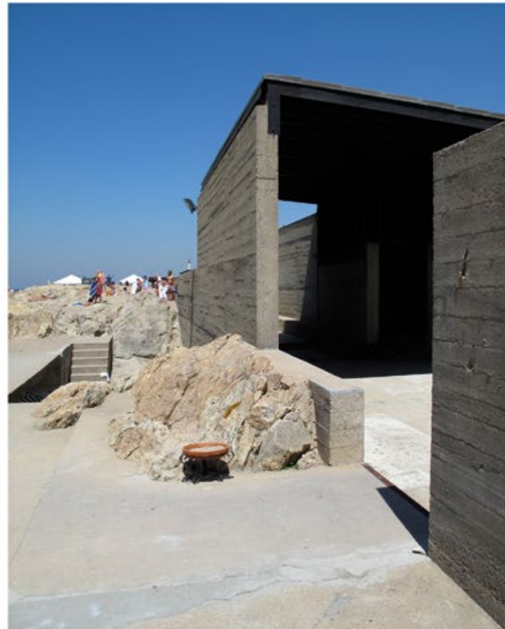
Figure 4.14- The building uses a robust concrete pallet shade lighter than the rocky outcrops to distinguish between the man made and the natural (Archdaily 2016).
