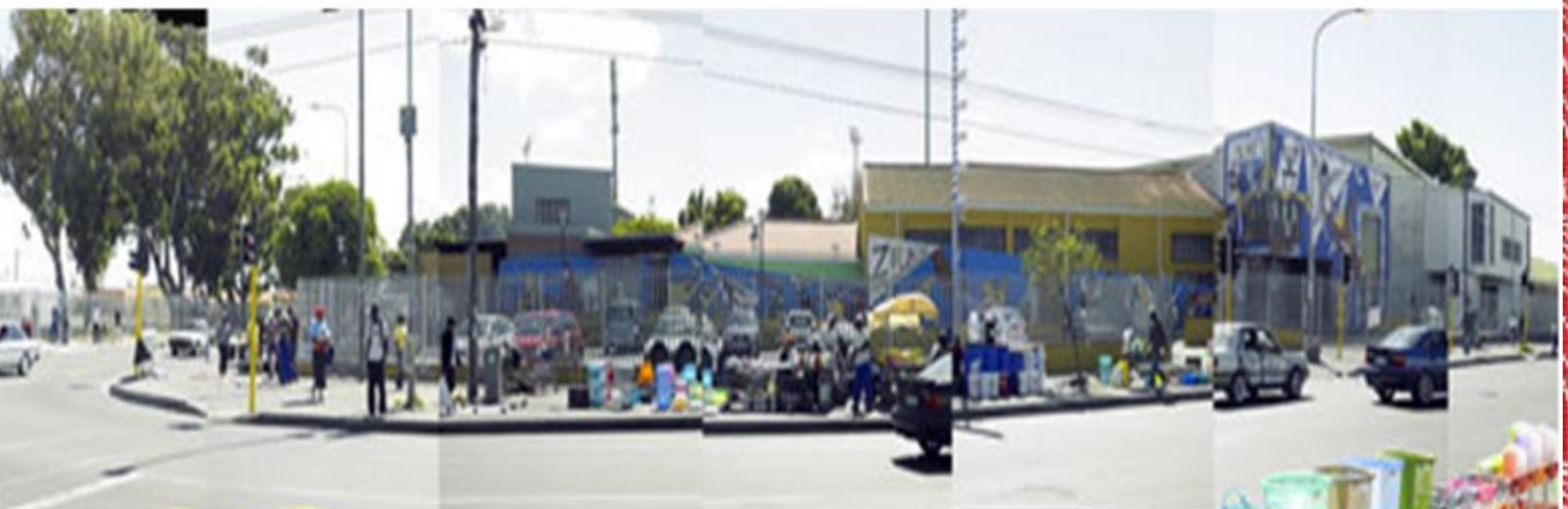
Figure 4.22 -Zolani Multi- Purpose Centre Operates from a very Intimate to a very Public Urban scale serving its community at different scales ( CSstudio 2002).
