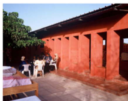
Figure 4.3 - Solid walls to protect the women with no openings except recessed entrance (Varanda 2004: 11).
