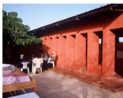
Figure 4.3 - Solid walls to protect the women with no openings except recessed entrance (Varanda 2004: 11).
