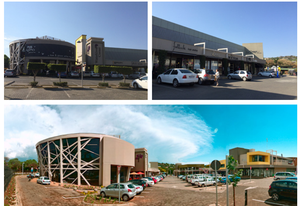
Figure 3.15. Waterkloof Corner Shopping Centre (Author, 2016; Advanced Building, 2012).
