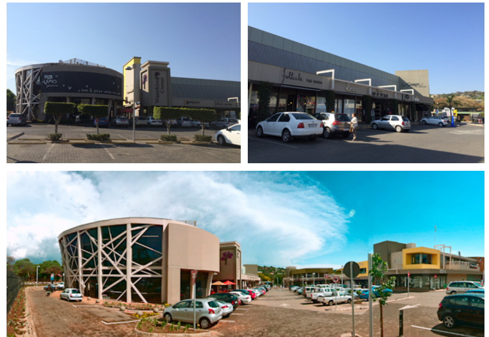
Figure 3.15. Waterkloof Corner Shopping Centre (Author, 2016; Advanced Building, 2012).
