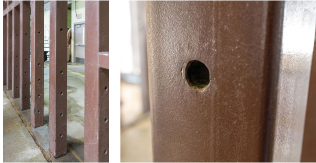
Figure 8.9 Left above: Circular steel members positioned diagonally, at the Elephant House in the Copenhagen Zoo. Figure 8.10 Left below: Circular steel members at the elephant enclosure at the Melbourne Zoo.
