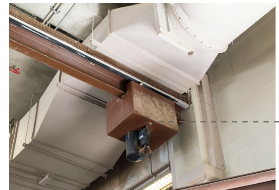
Figure 8. 7 Block and tackle running along steel beam used to raise elephants in emergencies, at the Smithsonian Zoo (Author, 2016).
