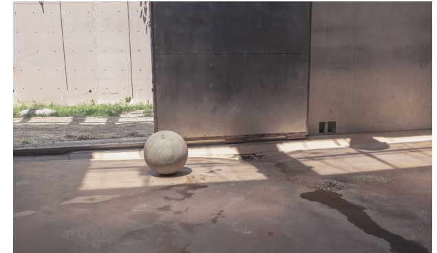
Figure 8.1 Rubber flooring in the elephant sleeping stalls at the Smithsonian Zoo, sloped to drain. Floors are routinely hosed down and disinfected to ensure a healthier environment (Author, 2016).
