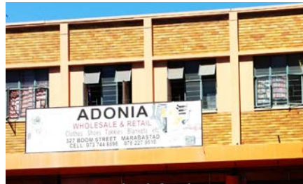
Fig.277. Existing brick facade.
