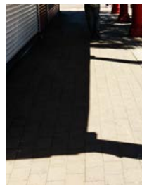
Fig.281. Existing concrete pavers.
