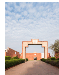
Fig.183. Entrance to the building.
