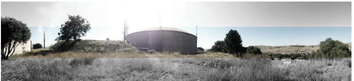
Fig. 71. Atteridgeville Reservoir - north.
