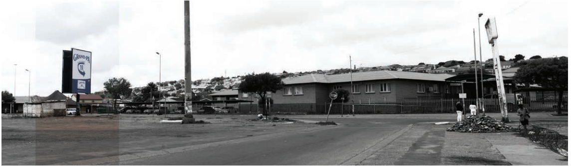
Fig. 46. Southern view of Atteridgeville Clinic on Ramohoebo
