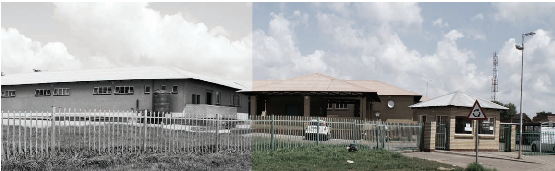
Fig. 43. Atteridgeville Clinic on Mareka street.
