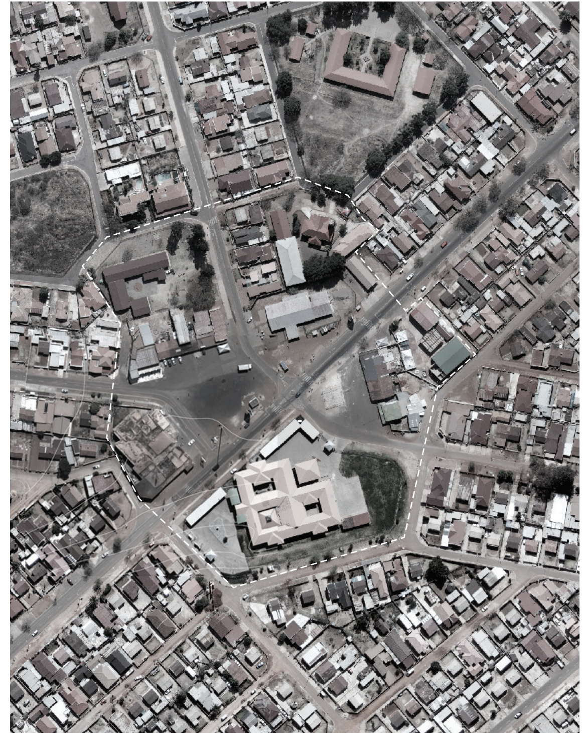
Fig. 59. Aerial photograph of Ramohoebo Square. (adapted from Tshwane GIS 2009). See Fig. 63 for key.
