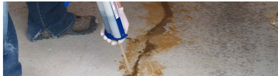
Figure 3.36. Caulking Repair of Concrete Crack (East Ronavtions, 2015)
