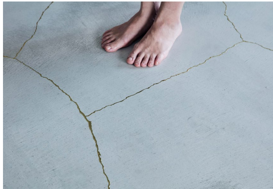
Figure 3.37. Gold Resin Infilled Concrete Cracks (Hasegawa, 2016)
