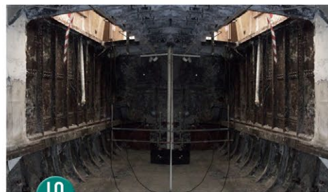
18 empty boiler room fore view
