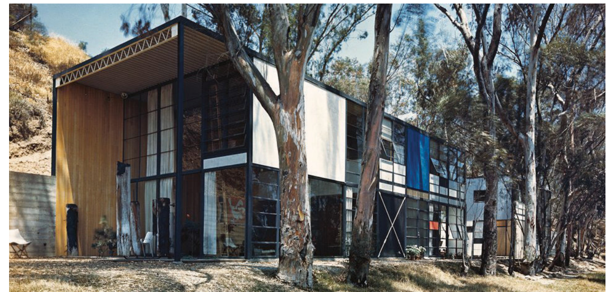
Left to right: 6.6 - Taliesin West (Archdaily, www.archdaily.com), 6.7 Rolling Huts and Delta Shelter (Archdaily, www.archdaily.com), 6.8 Tiny Diogene Hut (Archdaily, www.archdaily.com), 6.9 Case Study Houses (Lanonservancy, www.lanonservancy.org)
