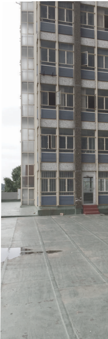
Figure 70: Rooftop event space at the Prinschurch building (Author 2016)
