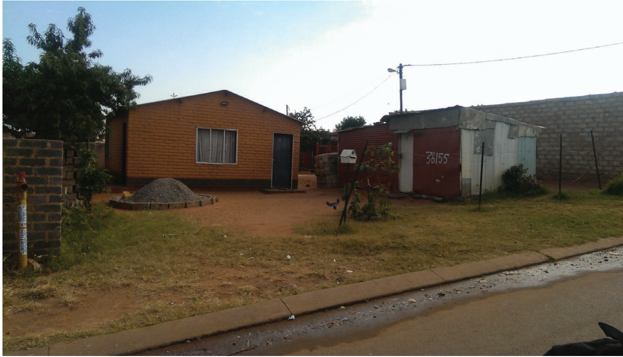
Figure 130: The RDP house and the shack, and the materials [Lusaka, Mamelodi] (Author 2016).
