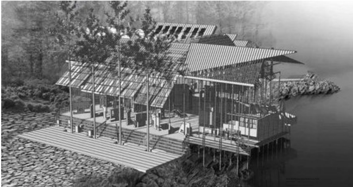
Fig 5.7 Aerial view of classrooms, also alongside a river (presidentsmedals.com, 2015)
