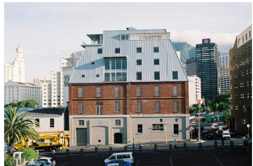
Figure 7_15 Building after addition [image online] available on: http://www.noeroarchitects.com/devilliers-hulme-office/ access on: 2016-10-04
