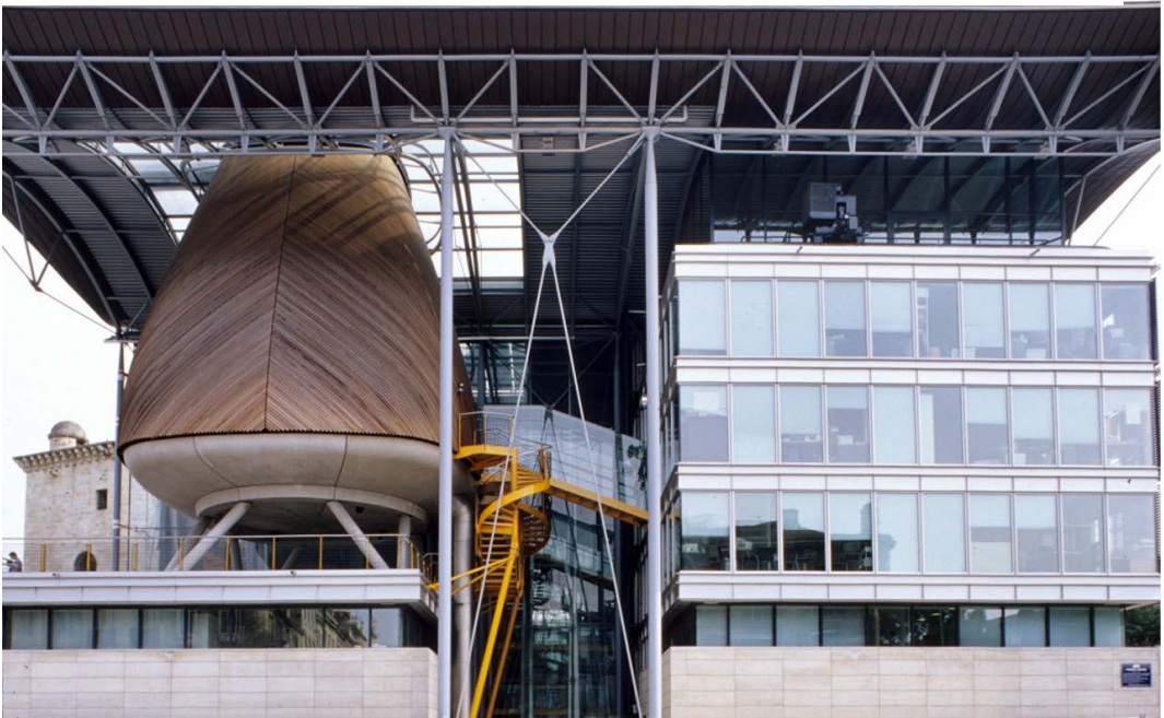
Figure 7_5 Bordeaux court in relationship to administration wing. [image online] available at: http://larryspeck.com/wp-content/uploads/2010/05/2009-0115.jpg access on: 2016-10-04
