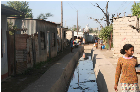
FIGURE 1: Poor drainage often causes serious floods in the informal settlements. Maintenance and infrastructure management are major problems as the municipal authorities devote their meagre resources to the formal city.
