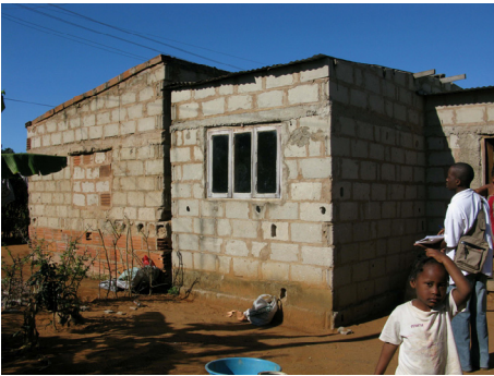
FIGURE 7: A typical dense informal settlement in Maputo with small modular units, each with a roof related to the length of corrugated iron sheets.
