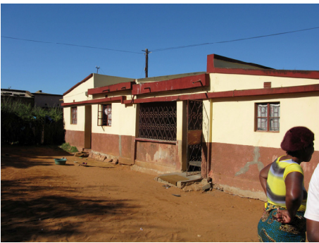
FIGURE 8: A modular small villa is the idea of a of the dream house for many residents in the informal settlements. The house has a veranda, two bedrooms and a sitting room. Kitchen and bathroom are separate units in the back yard (Quite wealthy families are also found in the peri-urban areas – often the architectural style of their dwellings will bear reference to the small Portuguese villa type).
