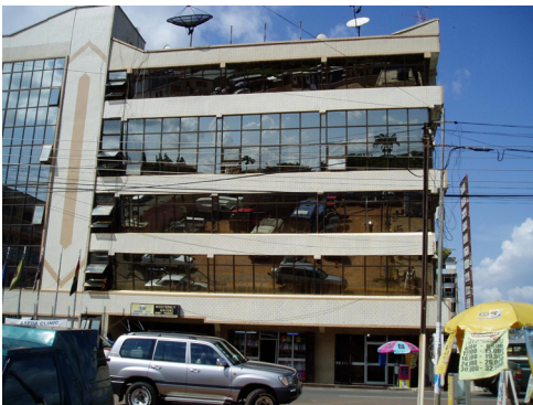
PLATE 2: A building constructed after complete demolition of an existing structure (Author).
