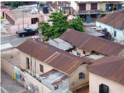
PLATE 3: A derelict building under threat of being gentrified (Author).
