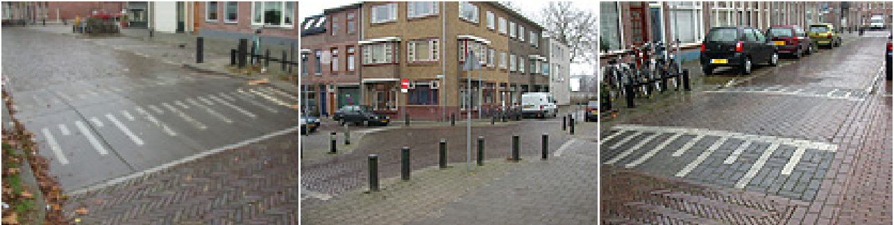
Figure 1: Typical traffic calming at access roads (30 km/h zone)
