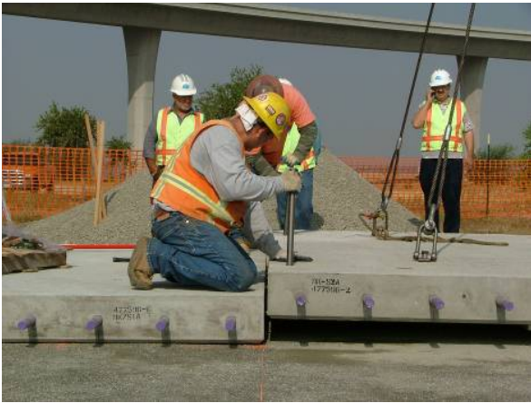
Figure 4. Precise placement of the slab on the sand bedding layer and hose with fitting for injecting grout
