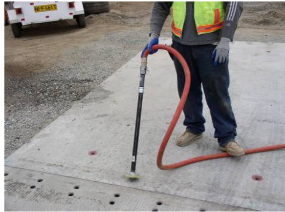
Figure 4. Precise placement of the slab on the sand bedding layer and hose with fitting for injecting grout
