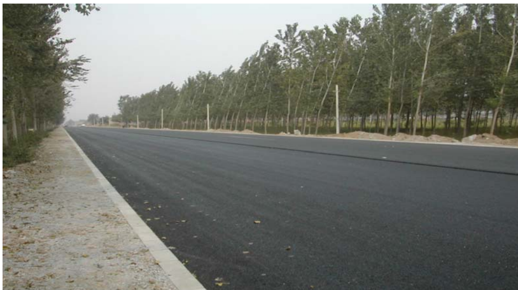
Photograph 4 – View showing the BRASO mix ( LHS ) and Porous Asphalt ( RHS )
