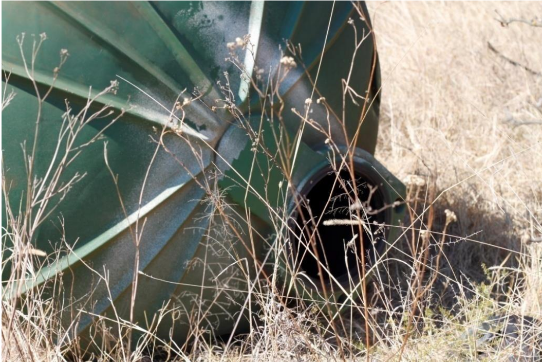
Figure 35: Water tank, 2011. Photograph by author.
