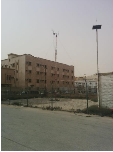
Fig. 4. Wind tower at Pearl beach
