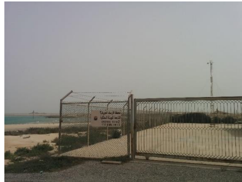
Fig. 3. Wind tower at Al-Bahar desalination plant
