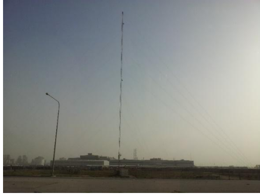
Fig. 2. Wind tower at Industrial area (Central)
