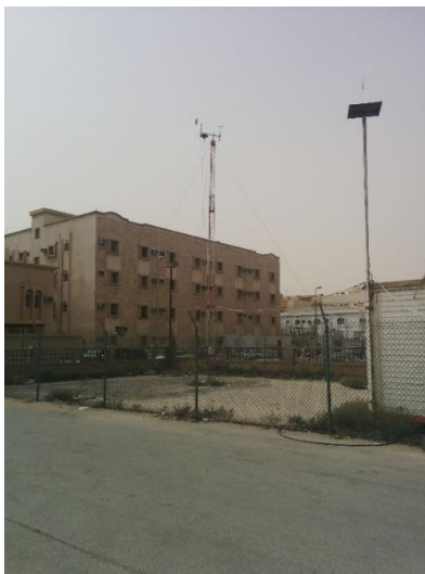
Fig. 4. Wind tower at Pearl beach
