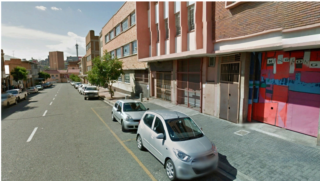
Figure 20: Street view of the King Kong Building, New Doornfontein Documentation, photograph Johannesburg, South Africa
